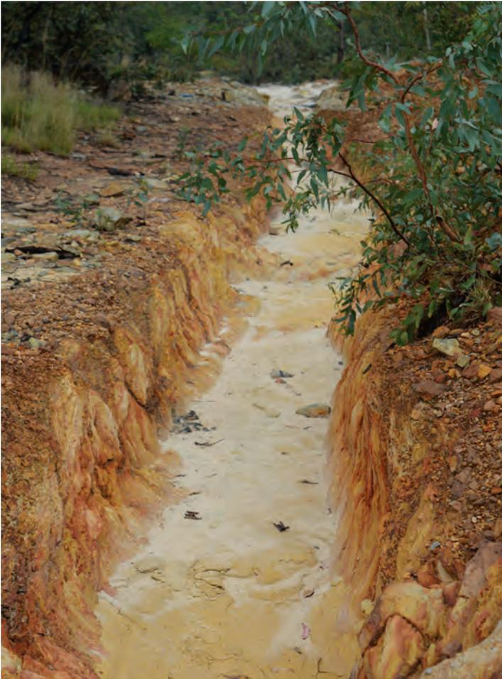
West Wits has also conducted trenching to expose shallow mineralisation on the Soweto Cluster
