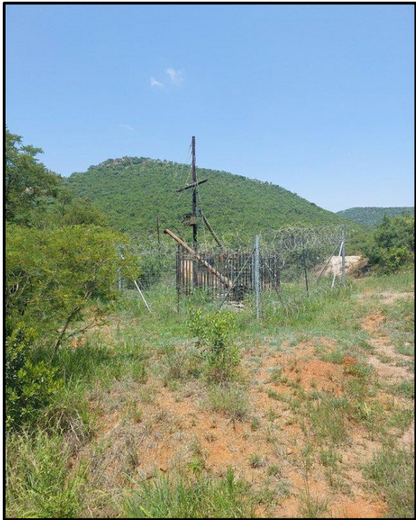
Figure 7.4. Existing infrastructure situated along the southern boundary of the application area .
