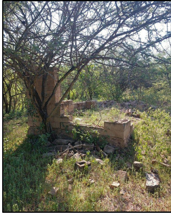
Figure 7.7. Ruin 2 - Partially broken-down structure situated in a thickly wooded area. The structure was built with cement bricks. Possibly part of past mining infrastructure.
