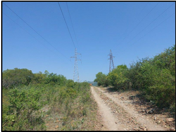
Figure 7.4. General site conditions along the powerline servitude
